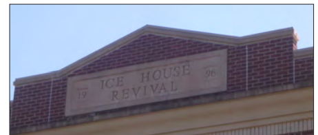
Masonry parapet sign
