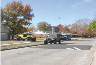
A concrete speed table on Norman's Vine Street is a calming device used to both slow traffic speeds and reduce volume.
