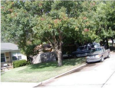
Curb and guttering makes a clear edge between public space and private space and improves drainage in some areas.
