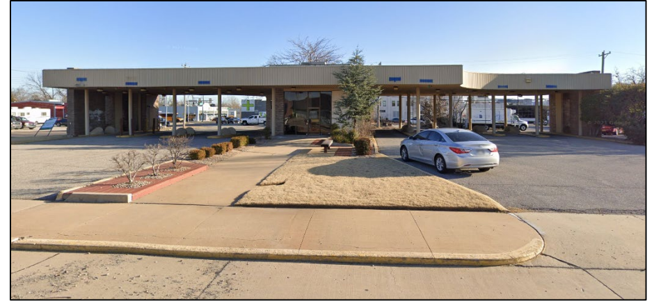
Current Exterior of 320 E. Comanche St
